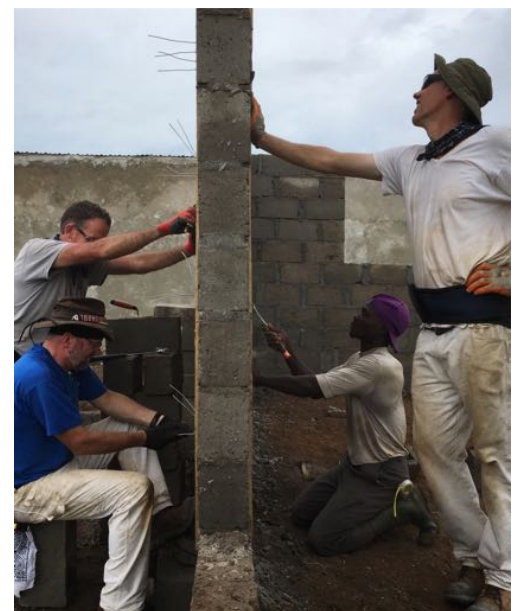
Below: Working together to tie a post.
